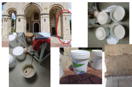
FIGURE 1. Application of newly developed bio-cleaning poultices on the Serbian Orthodox Church in Sremska Kamenica facade
